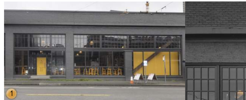
17FT WIDE BAYS WITH GEORGIAN FIXED WINDOWS, SAME TONE EXTERIOR MATERIAL AND WINDOW FRAMES.
