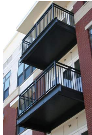
DECK AND RAIL CONCEPT: Project proposes a “fire-escape” aesthetic for the unit decks by detailing the metal stacked decks with expressed structure, exposed attachment detailing, and vertical stanchion metal railings.
