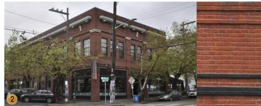
15-18FT WIDE BAYS WITH 2.5FT COLUMNS RED BRICK FACADE WITH DIFFERENT TONED WATER TABLE.
