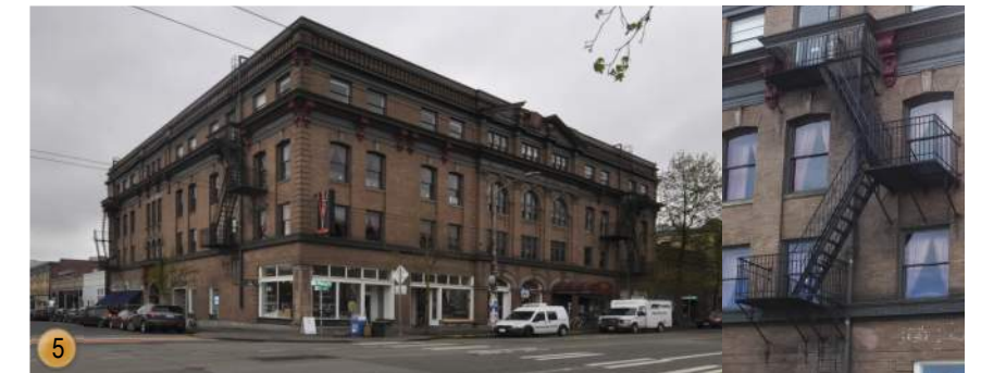
FLAT, RED BRICK FACADE WITH METAL DECKS 12-18FT WIDE BAYS AT RETAIL FACADE
