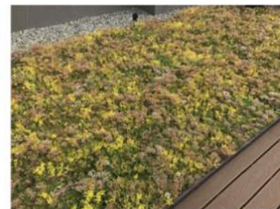
Green Roof - Sedum Mix
