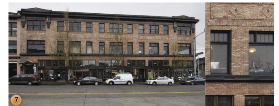
17-20FT WIDE BAYS WITH RHYTHMIC VARIATION OF FENESTRATIONS MULTI-TONED BRICK FACADE
