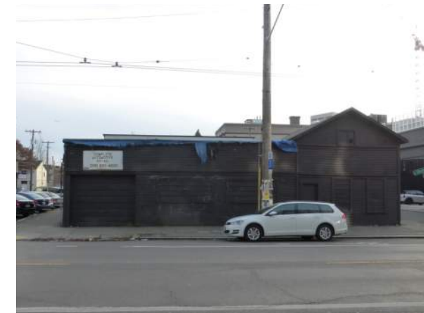
EXISTING BUILDING - E. UNION ST
