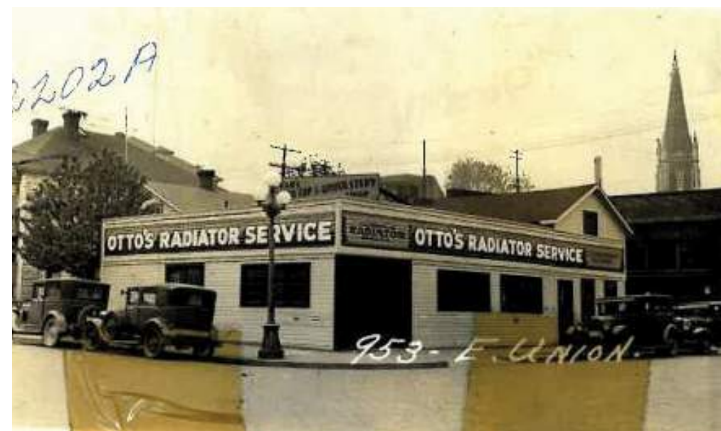
EXISTING BUILDING - E. UNION & 10TH AVE STREET FRONTAGE, CA. UNKNOWN
