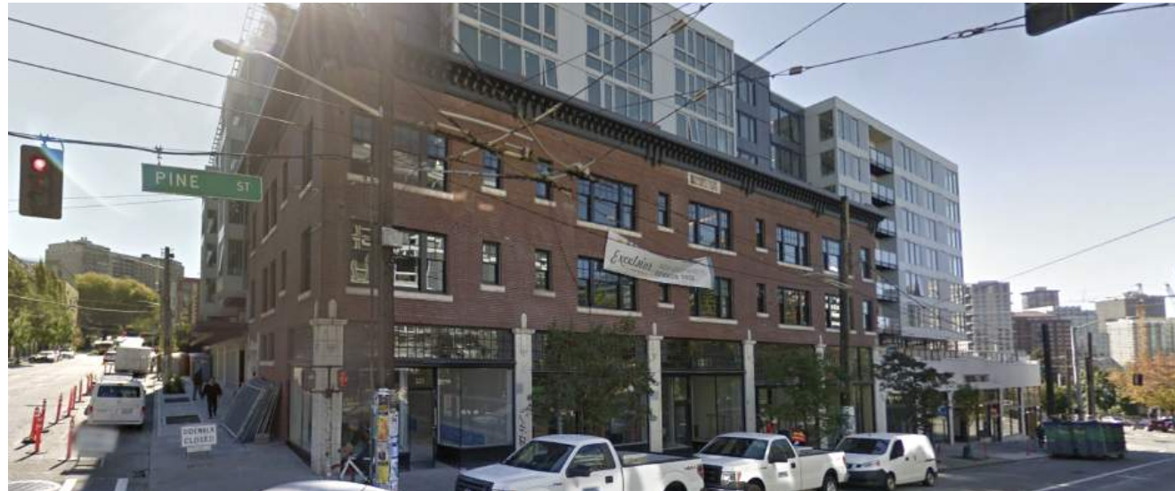
EXCELSIOR APARTMENTS: restored 1920's building with generous glazing at retail level
