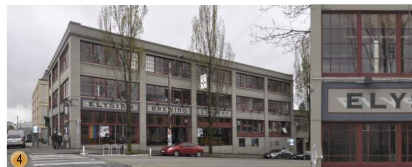
18-22FT WIDE BAYS WITH A SIGNAGE BAND BETWEEN GLAZING
