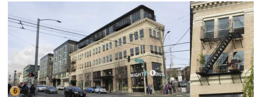
DOUBLE HEIGHT GROUND FLOOR. LIGHT BRICK FACADE WITH METAL DECKS STRETCHING ACROSS 3 WINDOWS.
