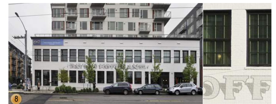
PAINTED BRICK FACADE AND SIGNAGE WITH PUNCTURED FENESTRATIONS
