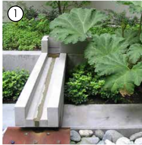
Runnel at downspouts
