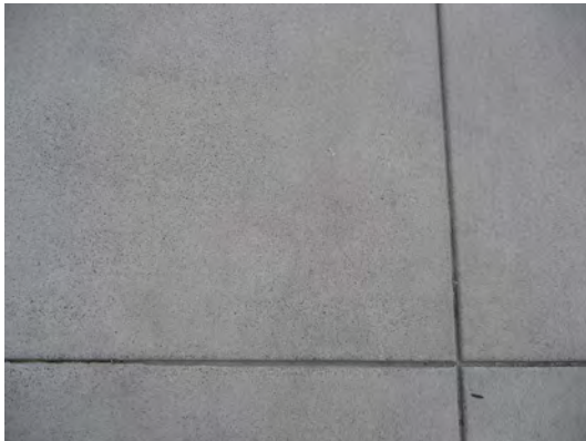
1 COS Sandblasted Concrete Paving with 2'x2' Score Pattern to match existing at Stewart Street
