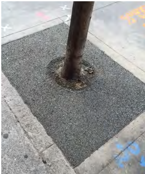
4 Flexi-pave Surfacing (At tree pit locations)
