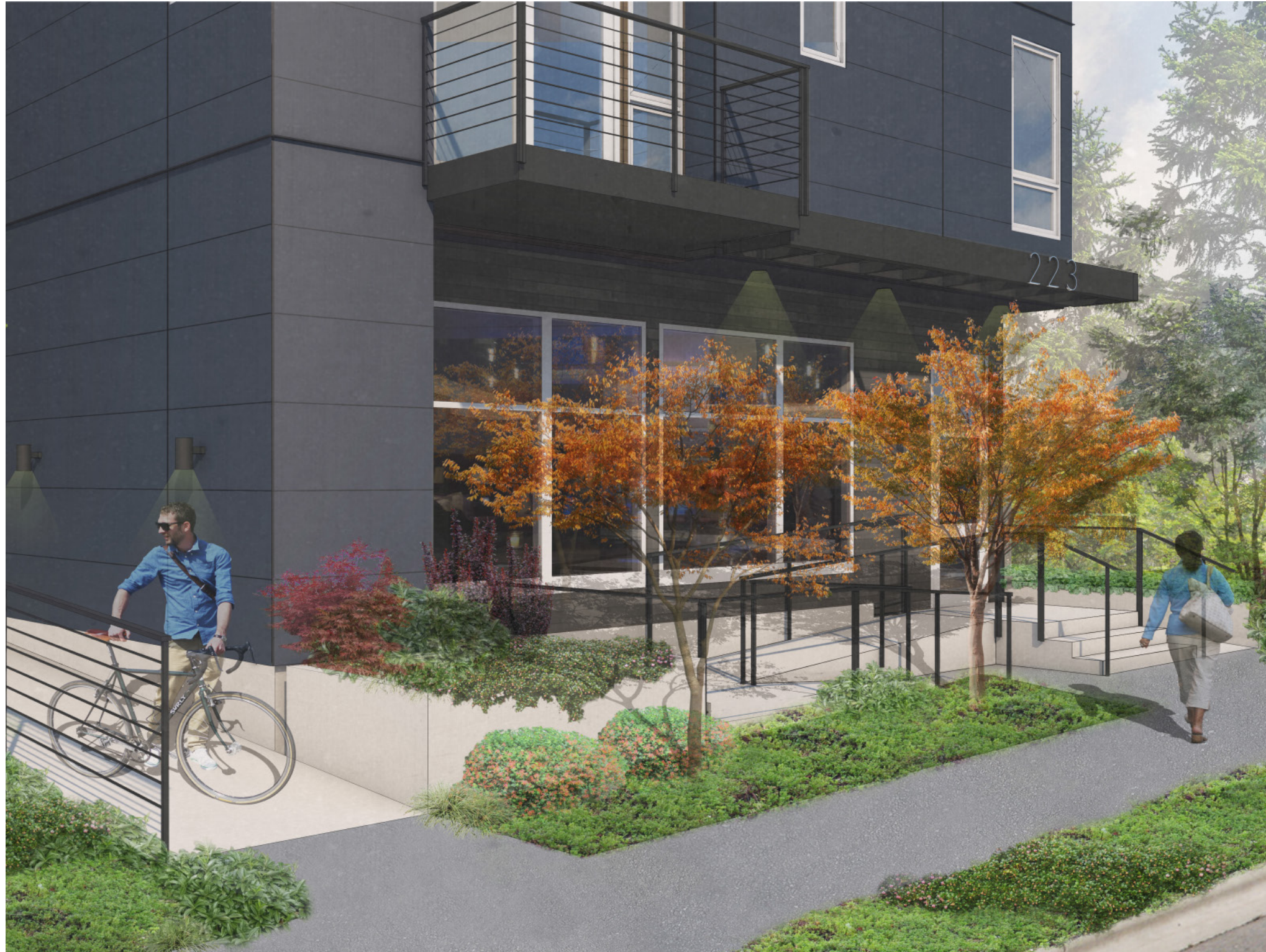
Street View looking Northwest
