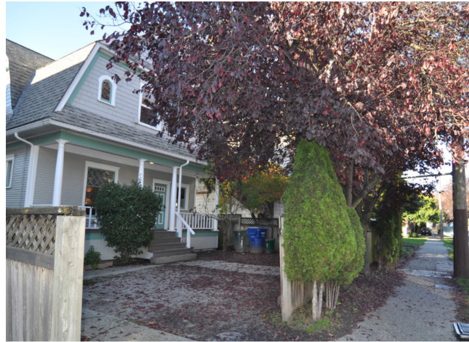
② View of site looking Northwest on 12th Ave. E.
