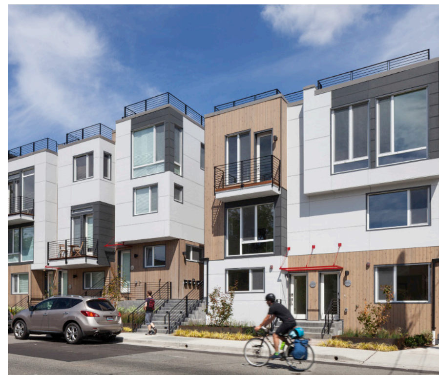
Townhomes at 414 12th Avenue E
