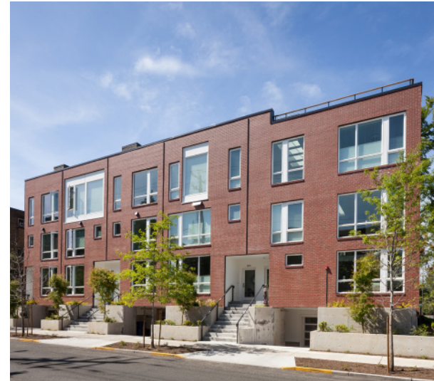
④ Mercer Rowhouses Built: 2016, 5 Units
