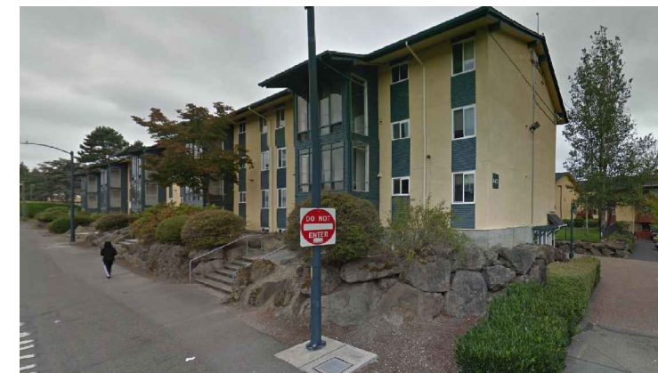
C 5952 MLK Jr Way (Apartments - 15 bldgs and 164 units)
