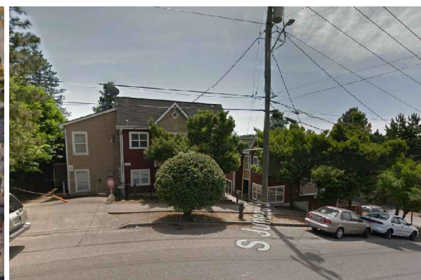
D 3801 S Juneau St (Townhouses - 2 bldgs and 10 units)
