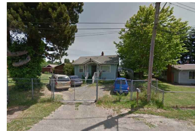
Single family #5944 facing 36th Ave S
