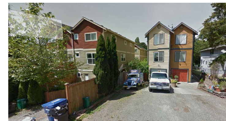
F 5937 36th Ave S (Townhouses - 3 bldgs and 3 units w/ 4bdrms) cross street
