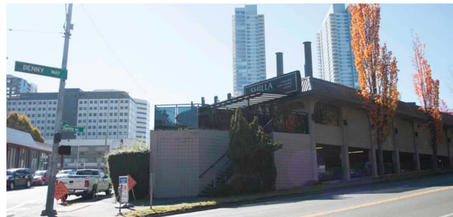
6 LOOKING SOUTH ACROSS DENNY WAY
