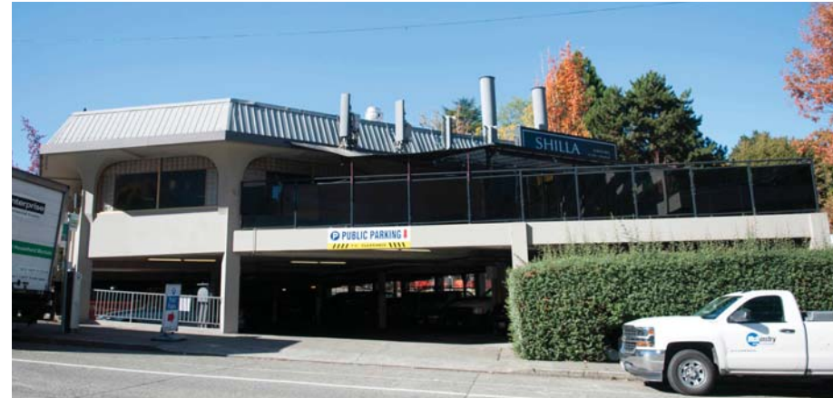
4 LOOKING NORTHWEST ACROSS BELL STREET
