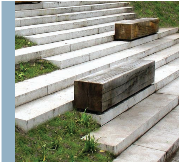
Concrete seat with heavy wood timbers
