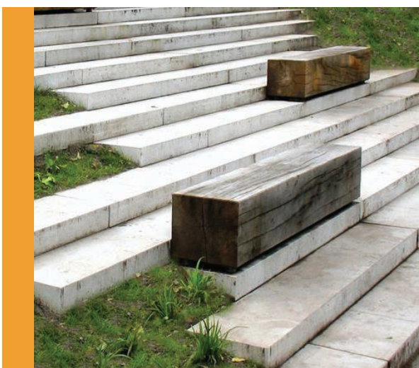
Concrete seat with heavy wood timbers
