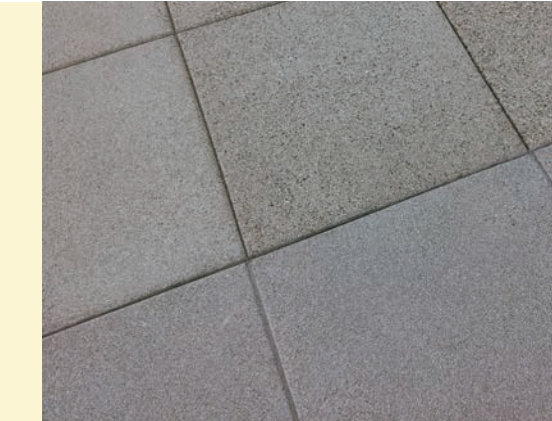
2' scoring with medium etched finish
