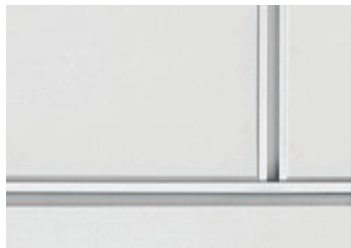
2 Fiber-cement Cembrit solid color panels, UV/fade resistant
