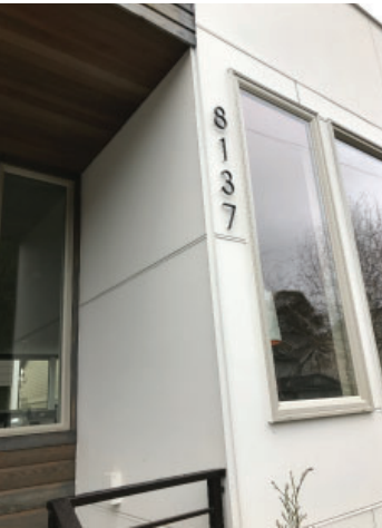
Cedar plank to FCB panels transition at the entry to the street level units with unit numbers
