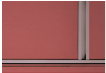
1 Fiber-cement Cembrit solid color panels, UV/fade resistant
