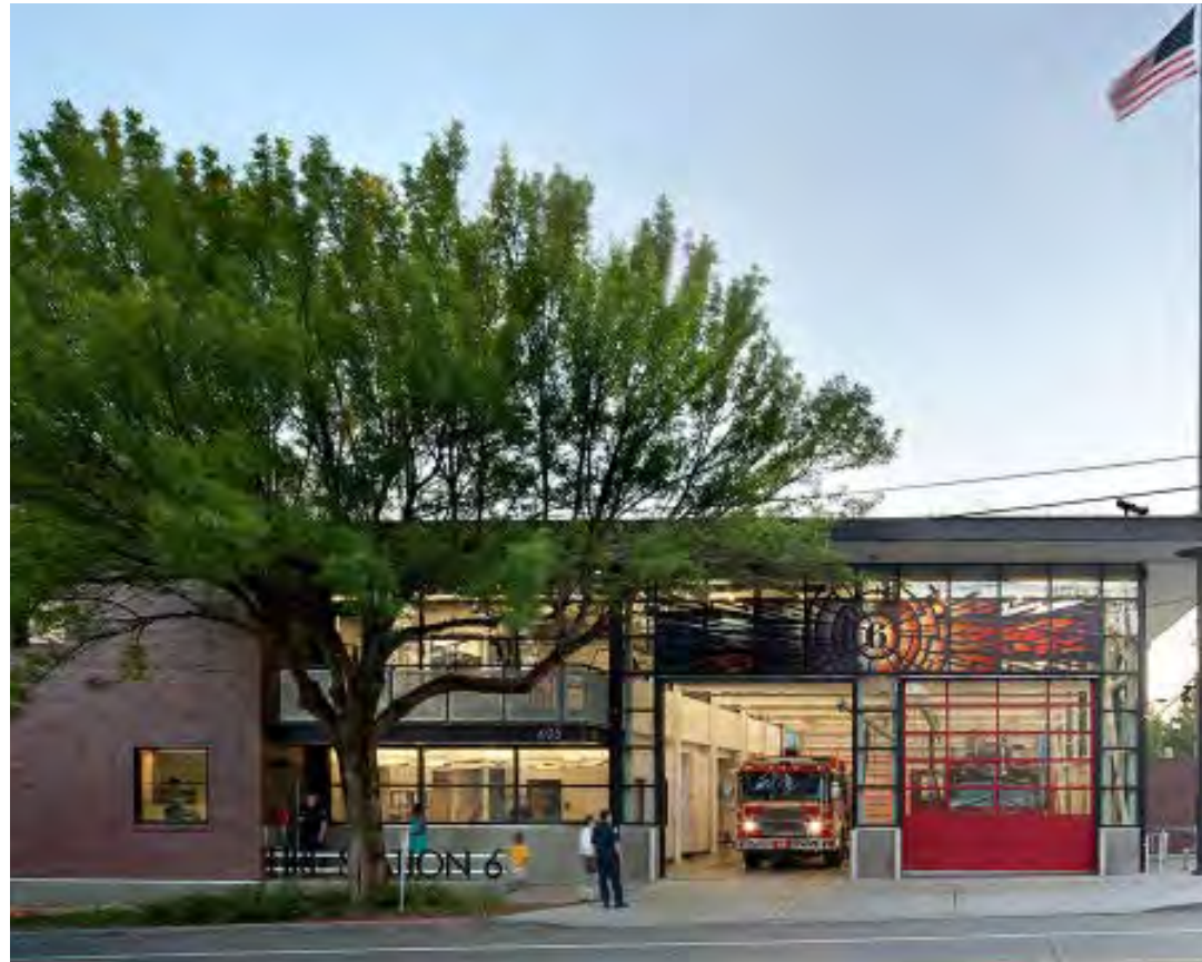
Seattle Fire Station 6 The material palette was guided by this building
