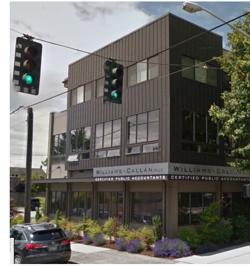
2 Metal Cladding on Mixed Use Building
