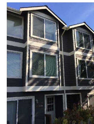
(C) 6624 Corson Ave S (Townhouse) neighboring project site
