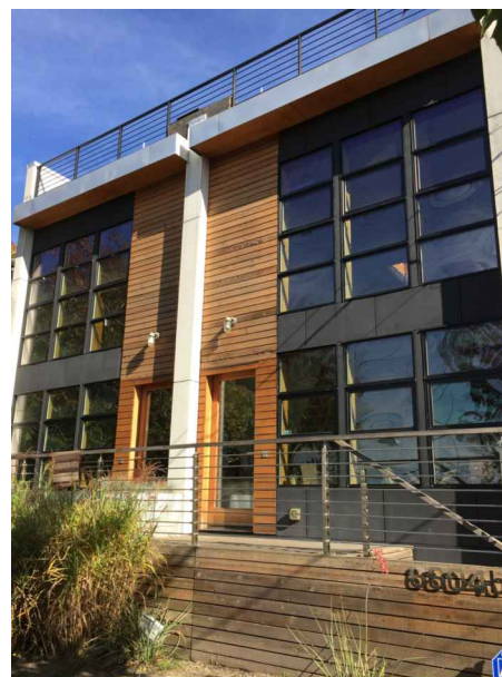
EXISTING SINGLE LOFTS ON NORTH OF SUBJECT SITE
