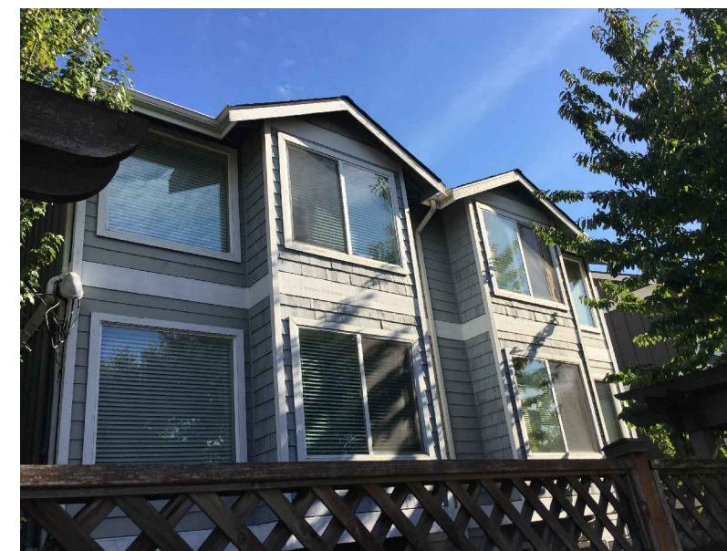
TOWNHOUSE TO SOUTH OF SUBJECT SITE
