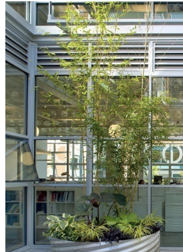
Storefront Curtain Wall
