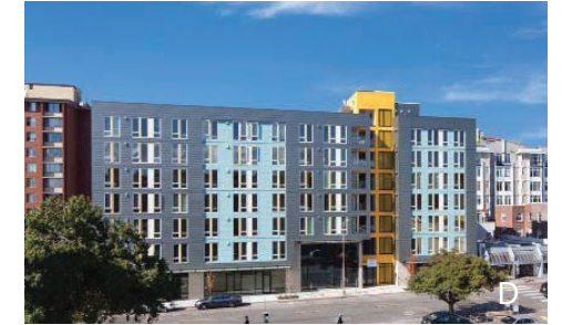
LIV APARTMENTS 4717 Brooklyn Ave NE 7 Stories Mixed Use 56 Residential Units
