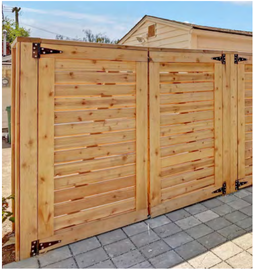
WASTE AREA SCREENED WITH HORIZONTAL CLEAR SEALED CEDAR SLATS
