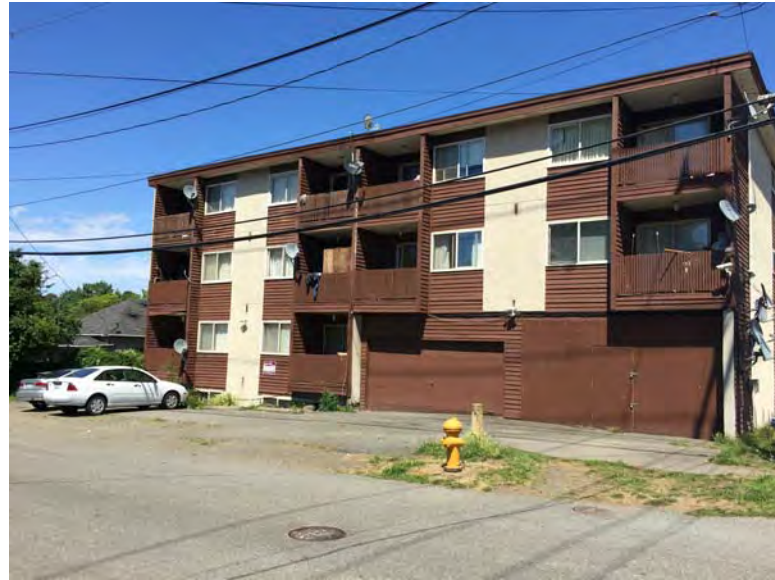
A - apartment building at 2900 S Byron St
