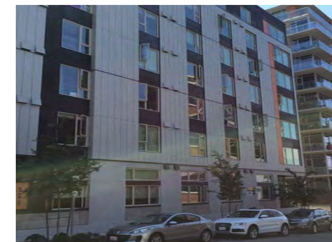
Example of vertical cement board panels in multi-family housing project in South Lake Union
