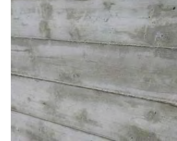
Board formed concrete at the base
