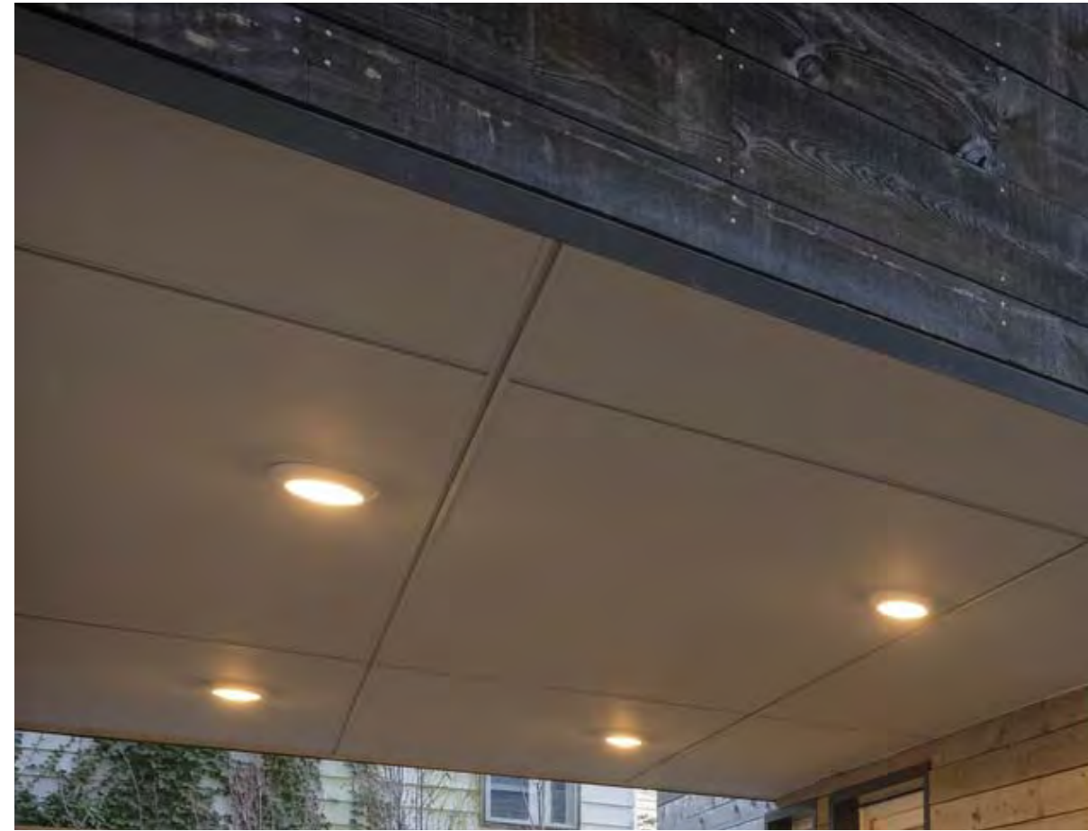
PAINTED FIBER CEMENT PANEL AT SOFFIT
