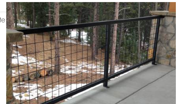
Metal Mesh Fencing
