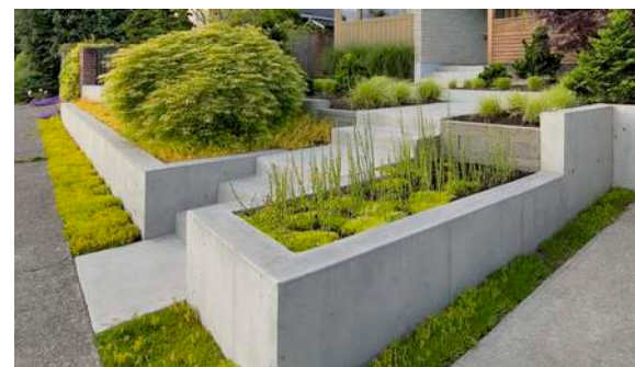
Raised Concrete Plant Beds
