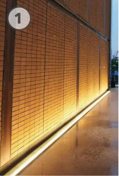
LED strip wall wash along perimeter
