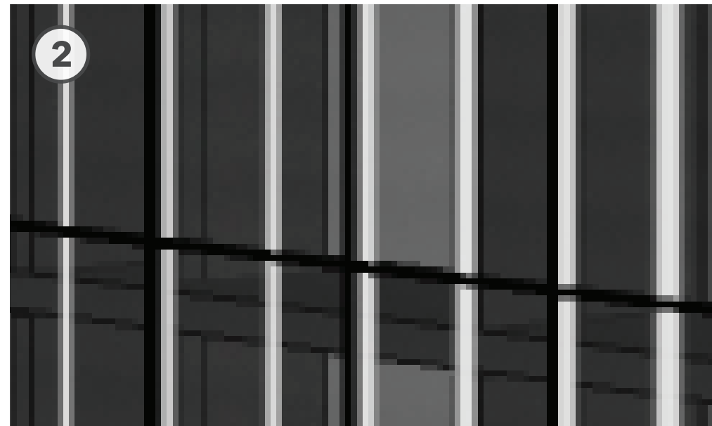
Detail of vertical lines - density of frit and height of vertical elements increase as they move away from the corner of Stewart and Minor. Density of reverse birch bark motif increases as density of vertical elements increase
