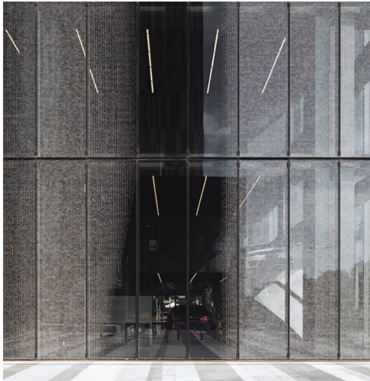
Landrover Office - Shanghai: pedestrian level experience
