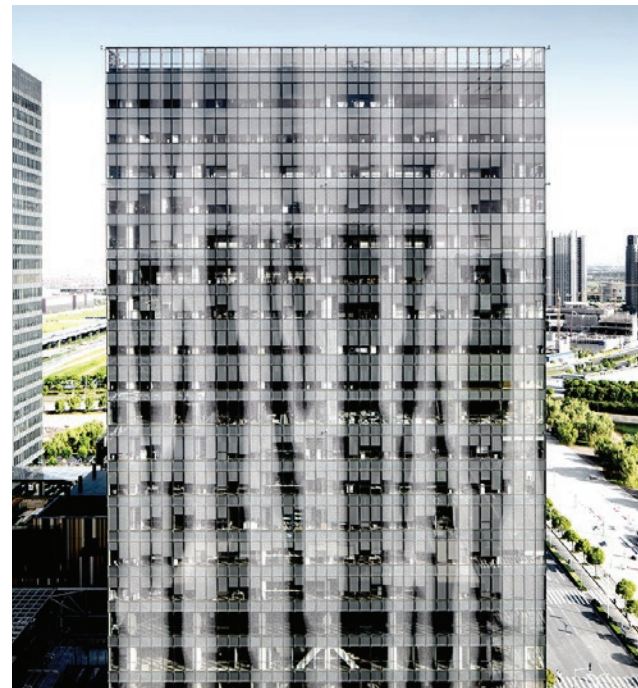
Landrover Office - Shanghai: frit facade pattern
