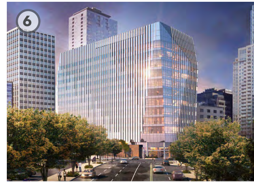
Seattle Children's Hospital - Stewart & Terry (under construction)
