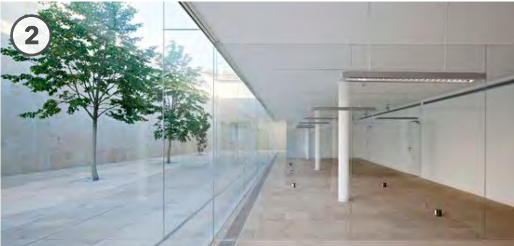
2 Silicone mullion curtain wall system to create high transparency
