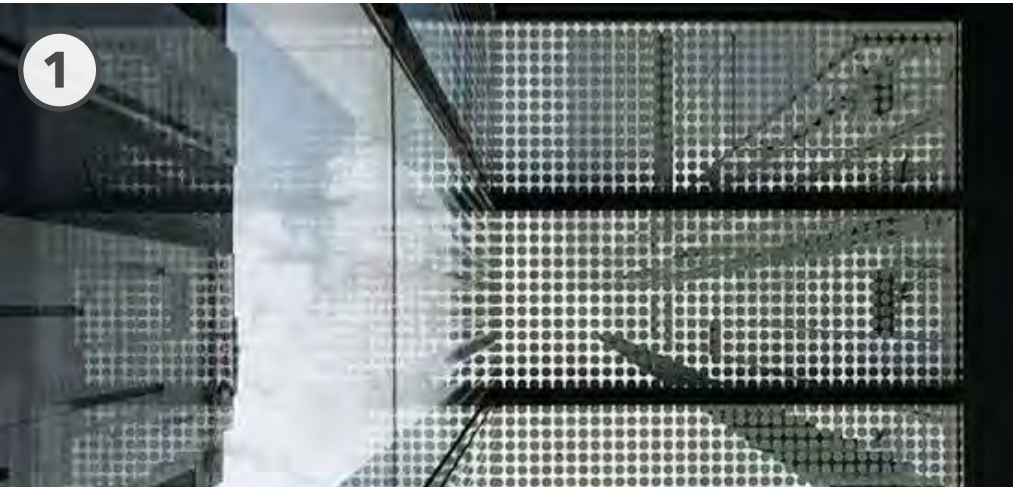
1 Unitized curtain wall system with frit pattern to create privacy and texture
