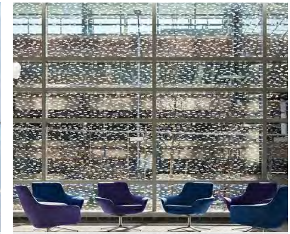
Interior view of patterned frit glass facade
