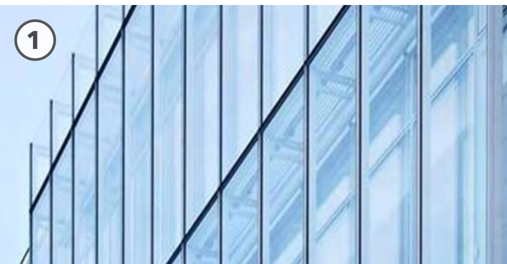
Unitized curtain wall with minimal silicone mullions and spandrel glass at slab
