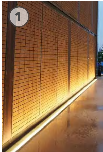
LED strip wall wash along perimeter
