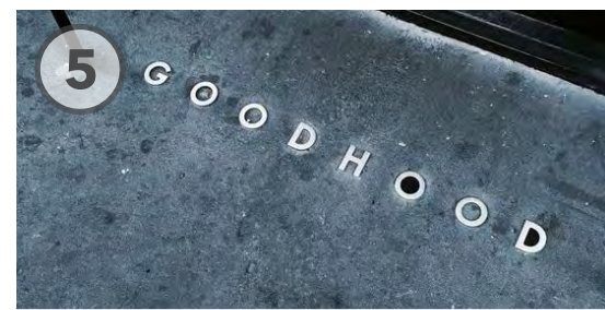
Concrete embed address signage
