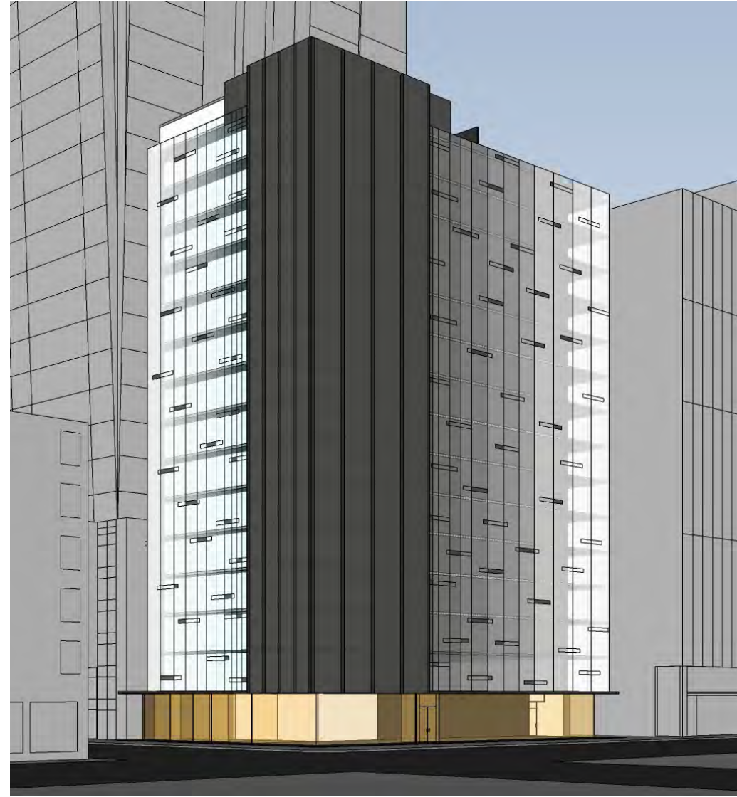
FRITT PATTERNED GLASS TO REPLACE METAL PANEL
