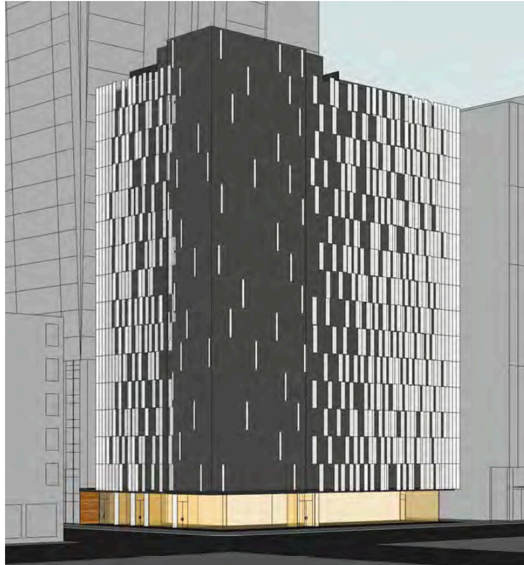
SCREEN SYSTEM PIXELATION ABOVE FLOATING BASE
