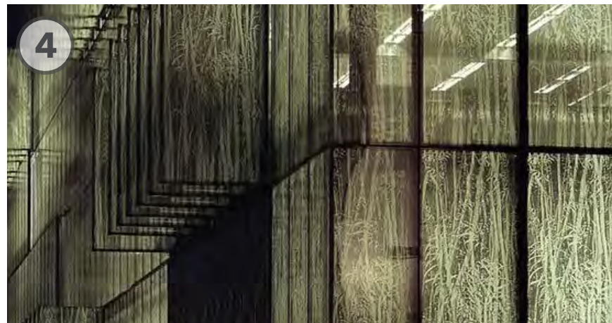
Backlit curtain wall with fritted glass
