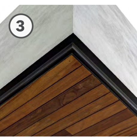
Wood panel soffit with c-channel edge
