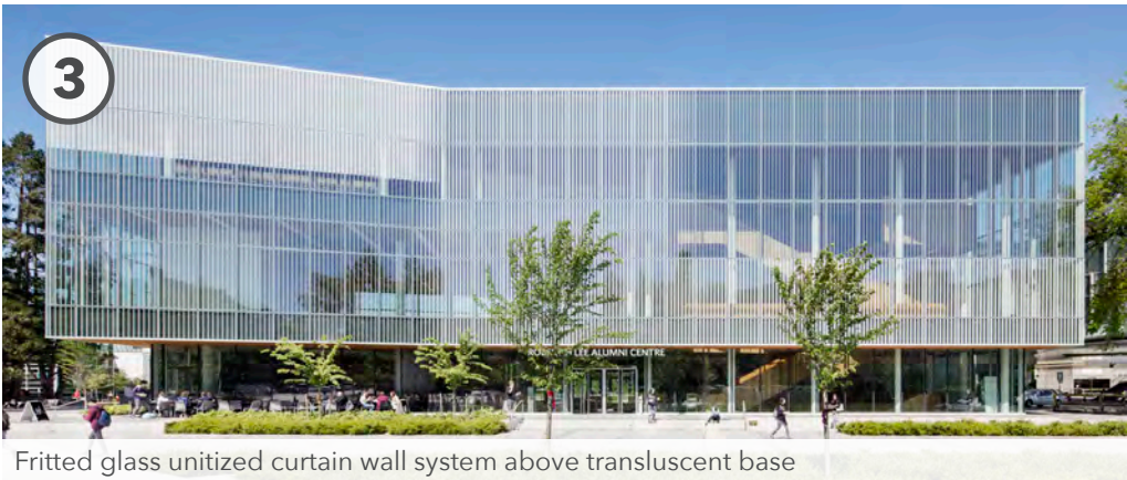
3 Fritted glass unitized curtain wall system above translucent base
