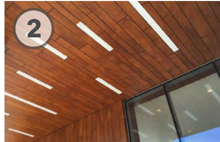
LED strip lights embedded in canopy
