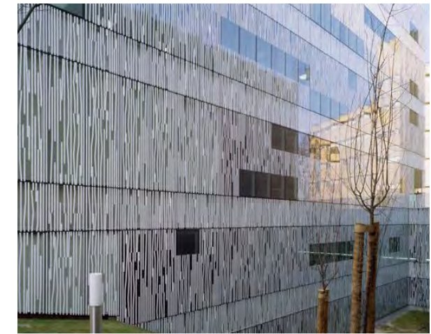
Texture created by frit patterning on curtain wall
