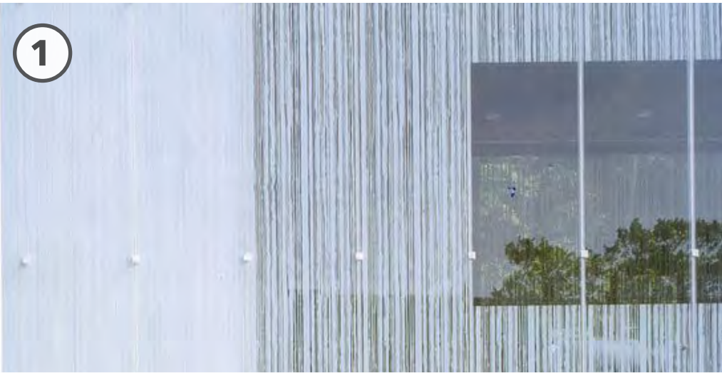
1 Unitized curtain wall system with frit pattern to create privacy and texture
