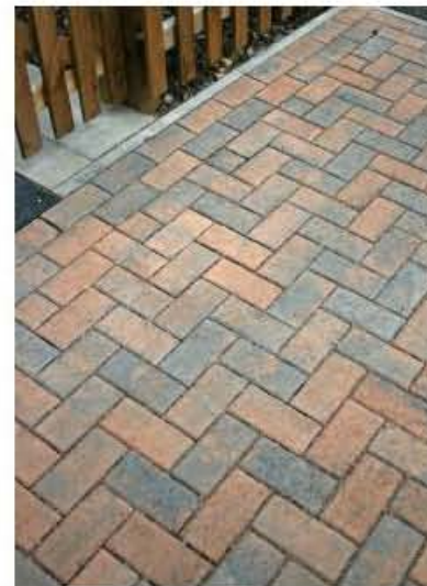
AQUAPAVE POROUS PAVERS IN COURTYARD AND WALK THROUGH PARKING AREA
