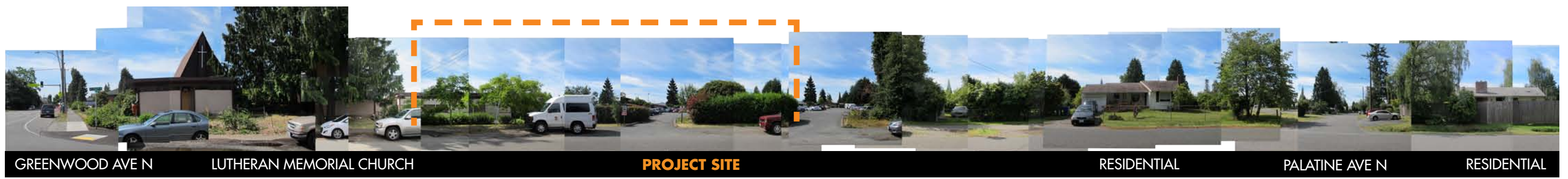
(D) N. 132nd St. (Looking South)
