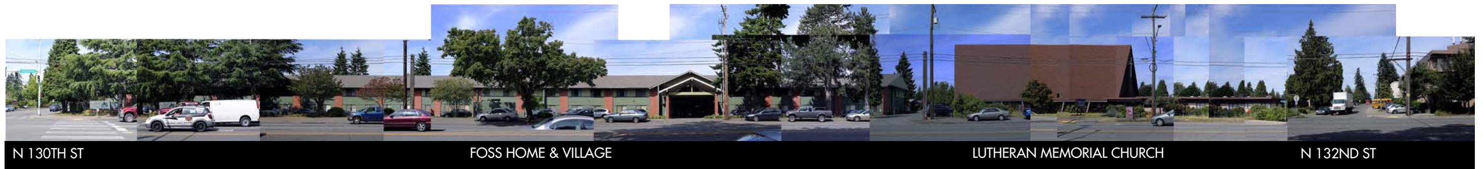
(B) Greenwood Ave. (Looking West)
