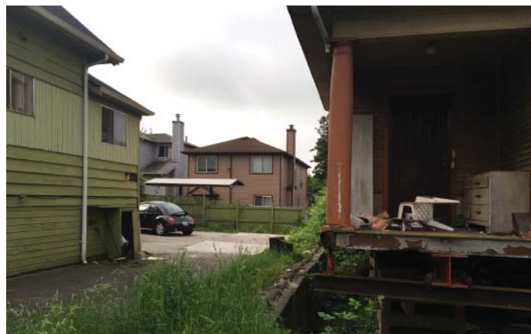
Structure 3 rear yard parking
