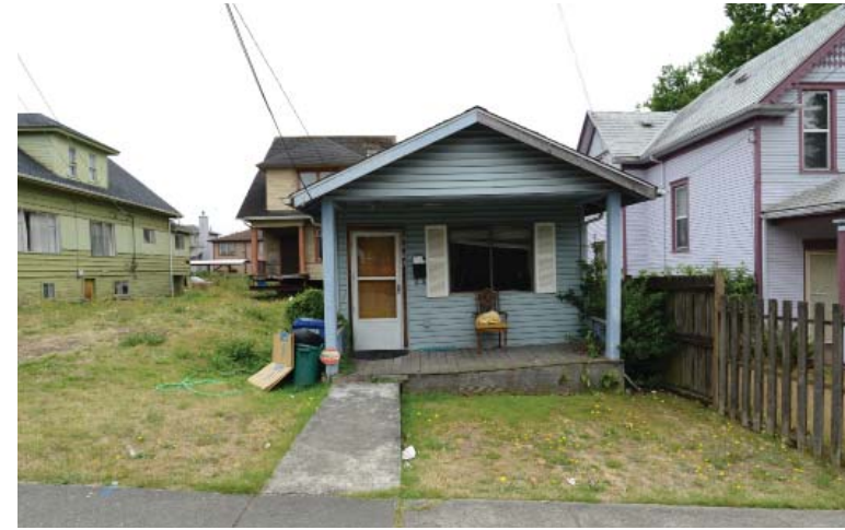
Structure 1 front porch north side
