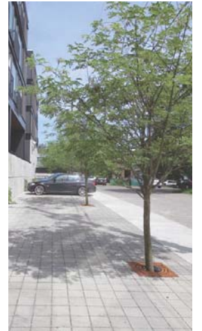
trees and permeable pavers
