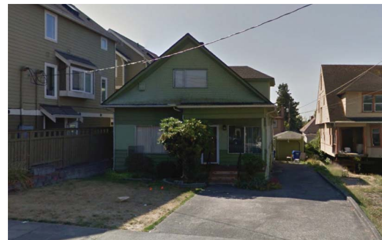
Structure 3 front porch north side
