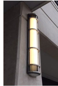
Exterior Wall Mounted Lights
