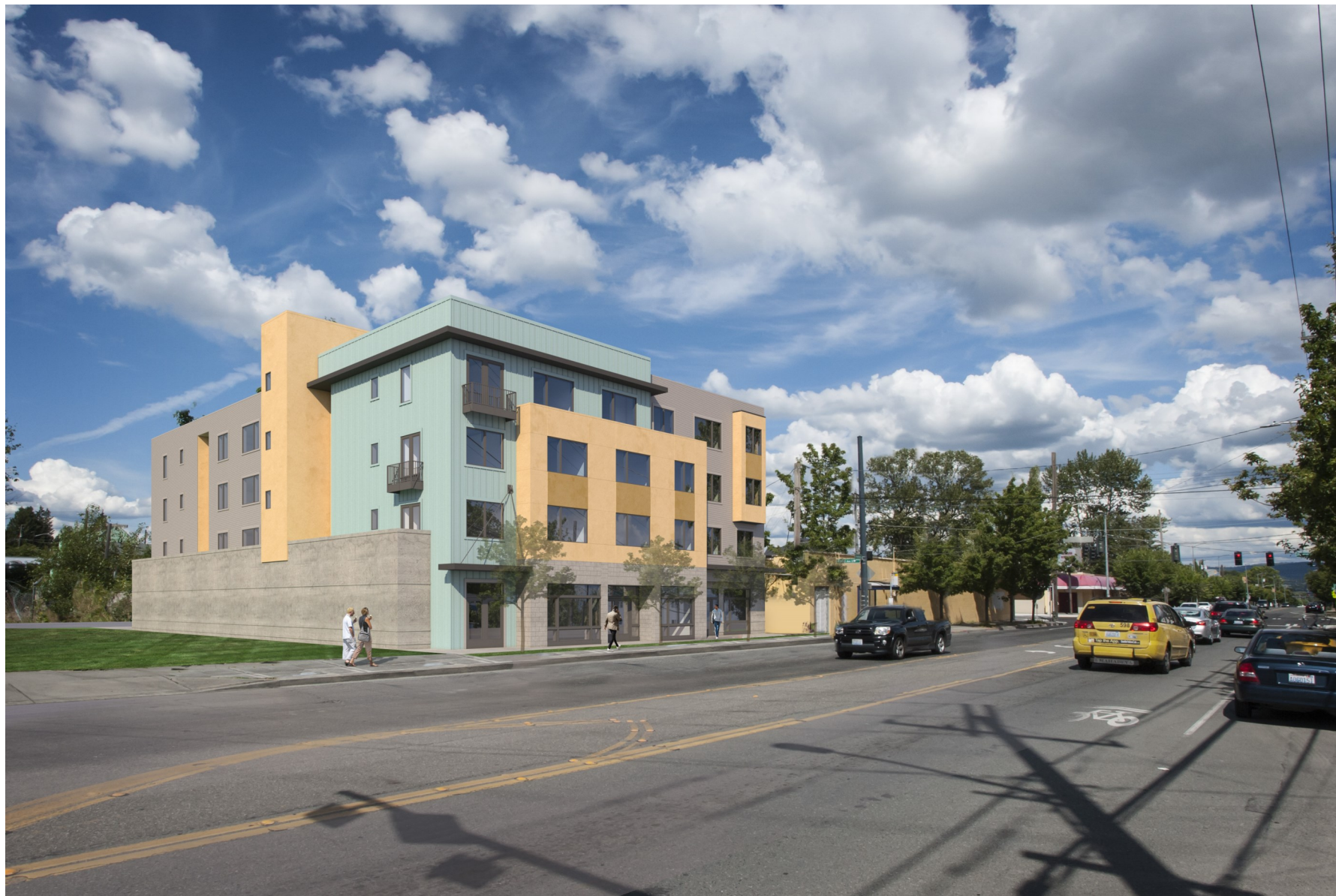
VIEW FROM HENDERSON STR. FACING EAST
