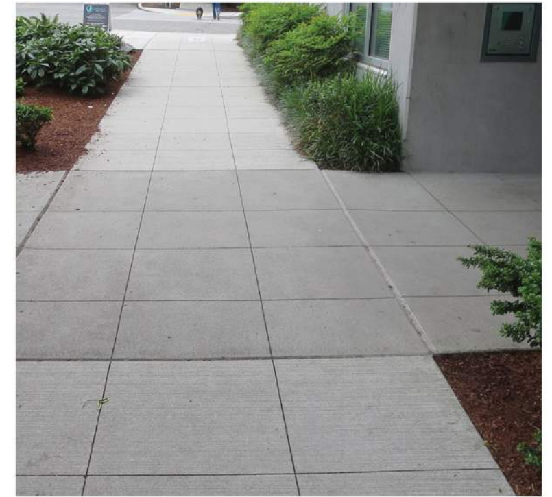
Paving: Light sandblast, deep tooled score joints
