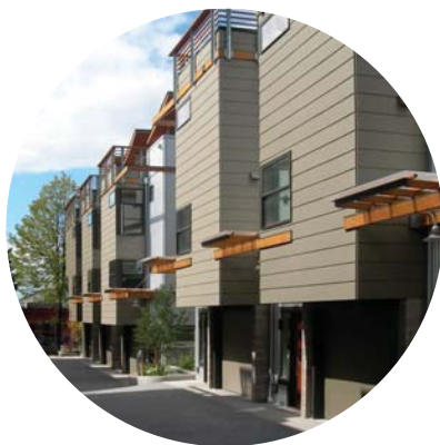
Townhouses on California Ave SW with Hardi-Plank siding
