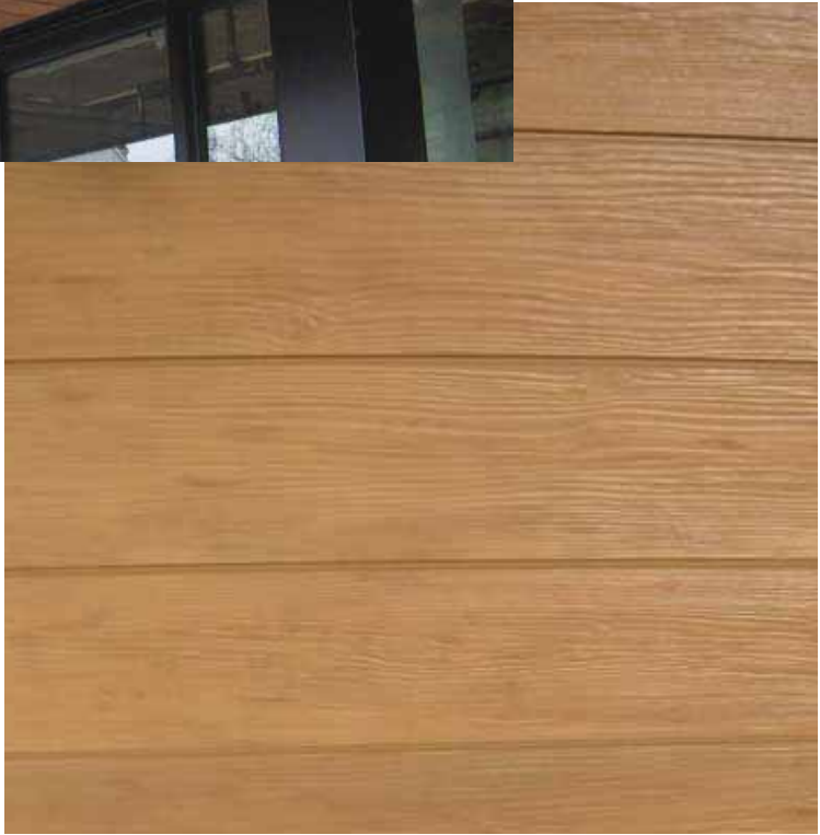
^ fiber cement board panel siding with the appearance of cedar
