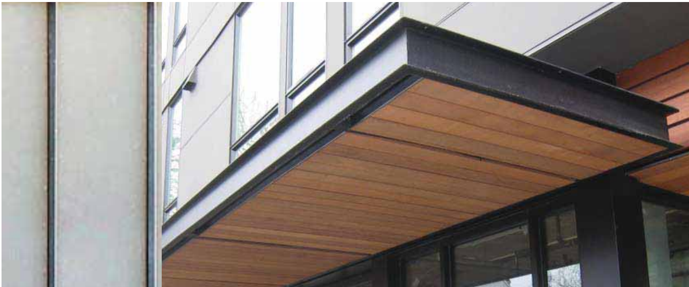
^ entry canopy with steel frame and cedar soffit
