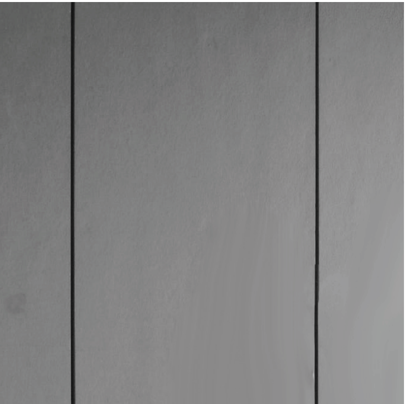
^ grey painted fiber cement board panel siding at stair towers
