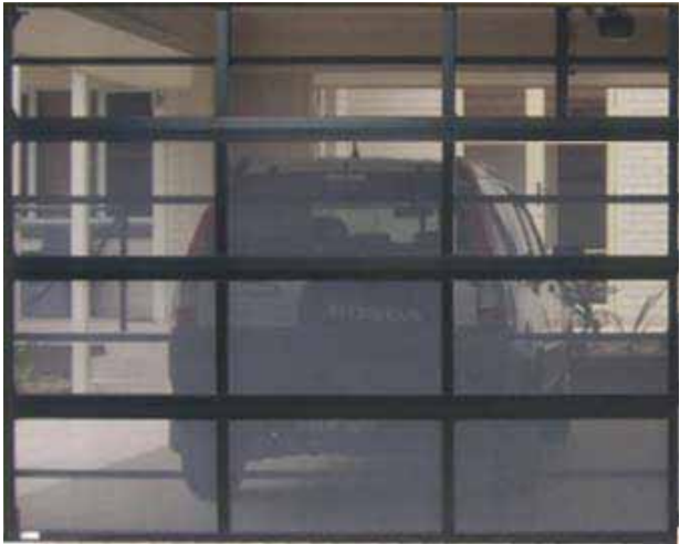
^ aluminum sectional door with metal mesh infill panels
