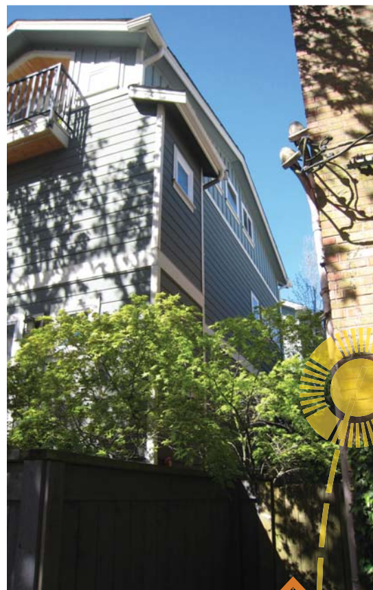
existing 3-story townhouse neighbor to the SW
