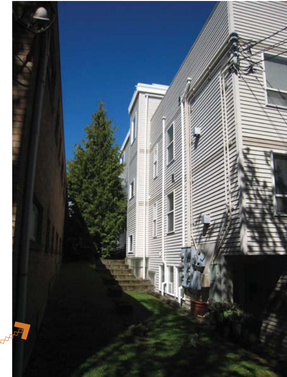
existing 3-story apartment to the east
