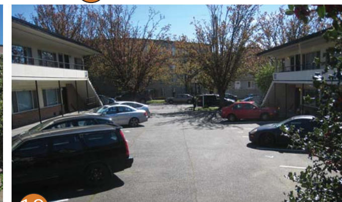
10 alley looking into site (east)
