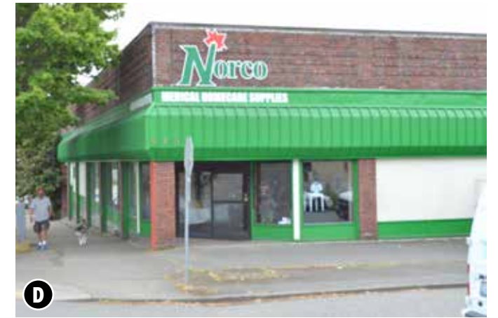
D Existing Use: retail, with jarring addition to historic brick building
