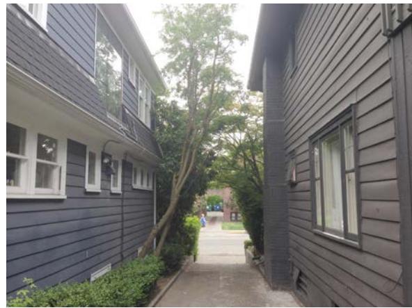
Existing driveway condition looking west
