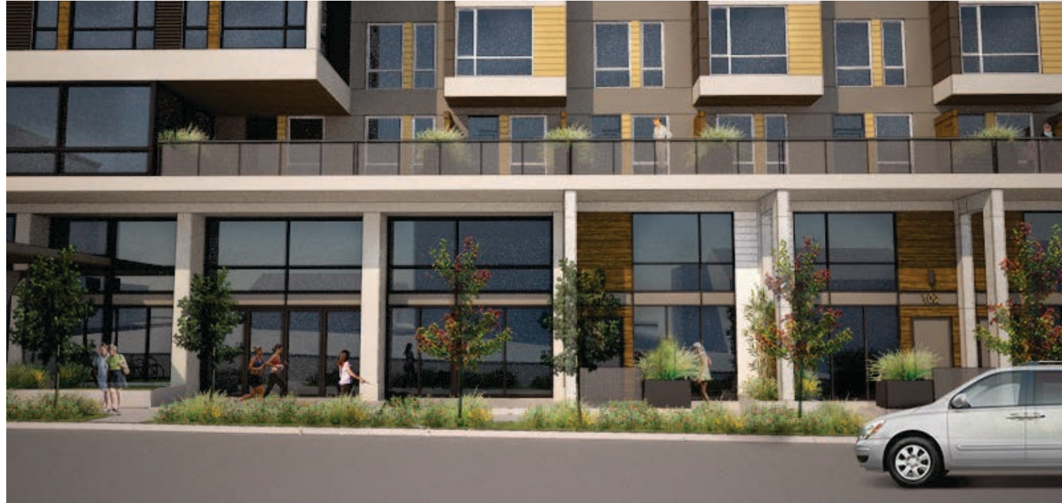
Valdok Ballard - Currently Under Construction Two Story Facade With Deck Above
