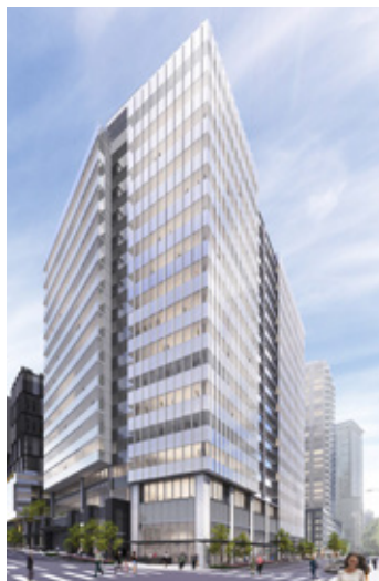
10 WSCC Expansion – Office
