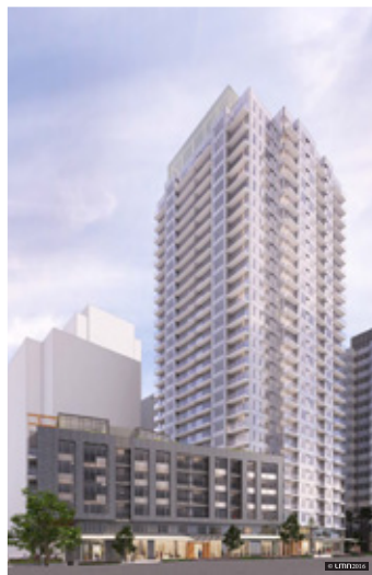
11 WSCC Expansion – Residential
