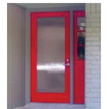
RAILINGS AND WINDOW FRAMES Black.
