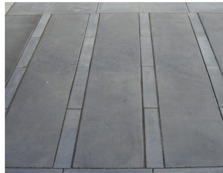
LINEAR CONCRETE PAVING AT ENTRIES
