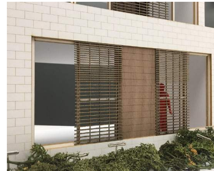
Pultruded fiberglass operable screens at 12th Ave
