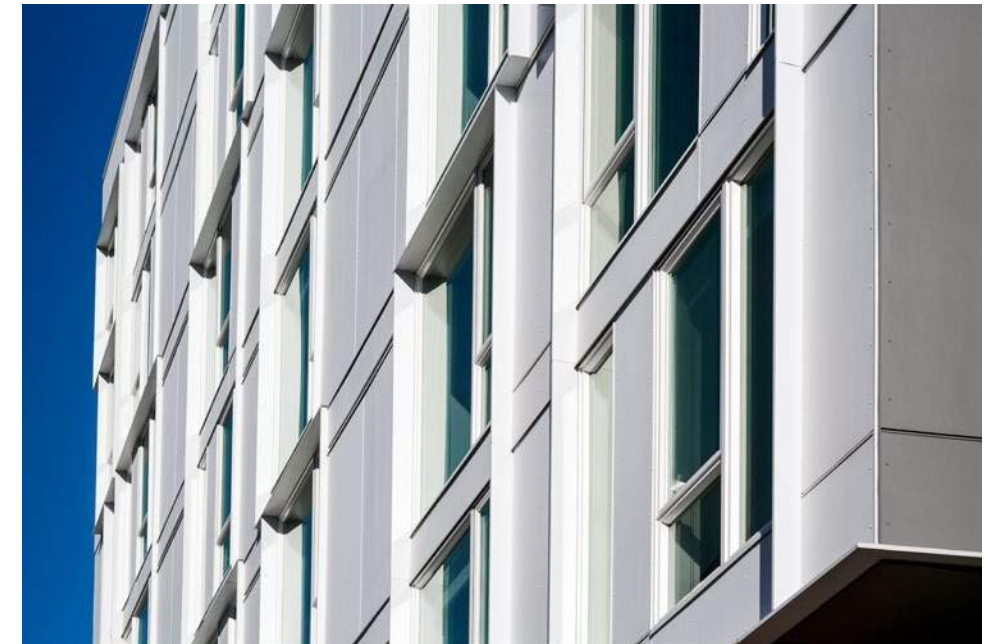
Cement Panel and vinyl window detailing at 8th and Republican.
