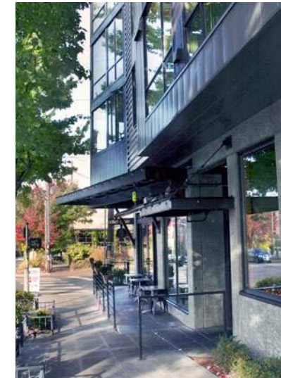
RECESSED CORNER ACCENTED WITH SEATING
