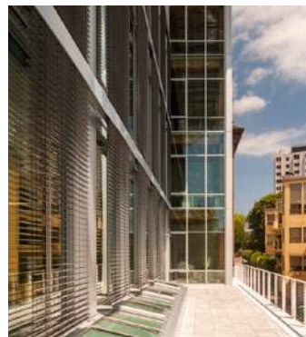
EXTERIOR SOLAR SUN SHADE
