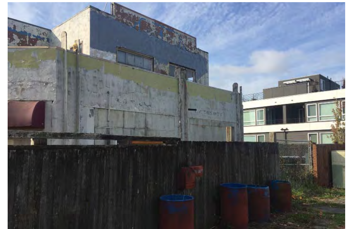
4 Looking SE from sidewalk at S Judkins St
