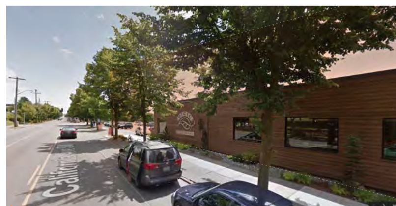
B VIEW ALONG CALIFORNIA AVE LOOKING S
