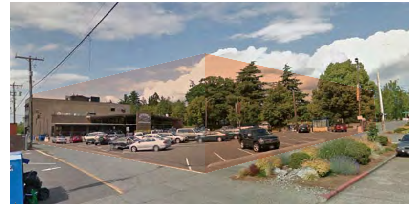
E VIEW FROM SW CORNER LOOKING NE
