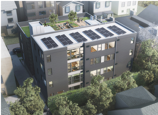
eastern - rear facing - facade dark grey lap siding with white cement board gasket and elev. shaft
