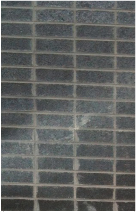
Brick - Stack Bond - Slimbrick Mutual Materials - Architectural Series Color: Coal Creek - Grout: Dark
