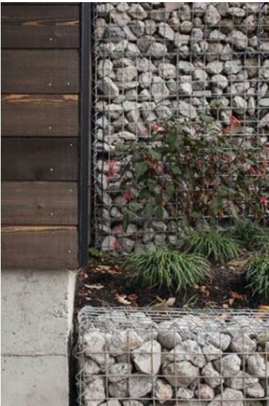
Integration of Gabion walls, concrete, cedar siding
