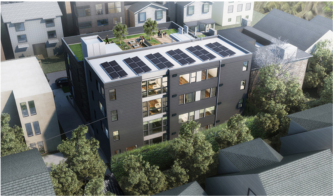
Horizontal Lap siding at rear of the building to correspond with residential materiality towards the east
