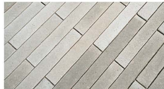
9. Permeable Paver Pedestrian Walk Way
