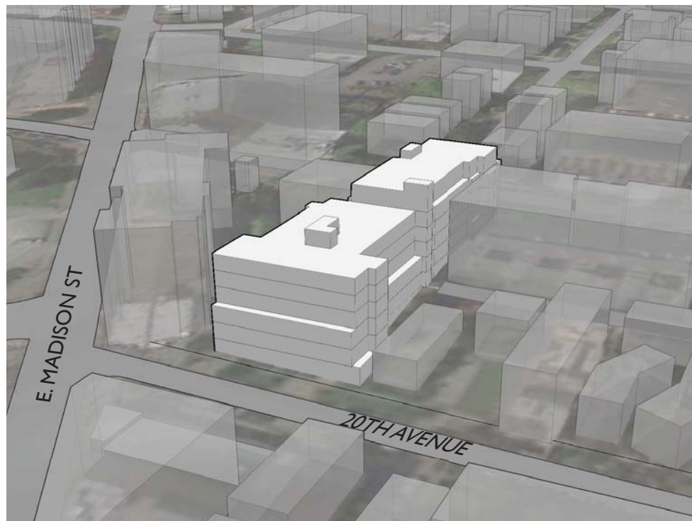
AERIAL VIEW LOOKING SOUTHWEST TOWARDS SITE
