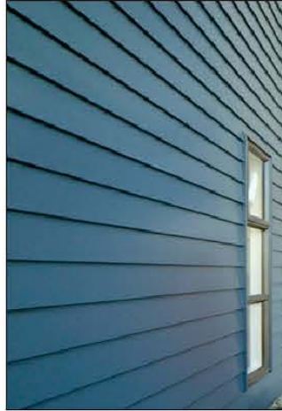
CEMENTITIOUS LAP SIDING ON THE BUMP-OUTS AND CIRCULATION TOWER
