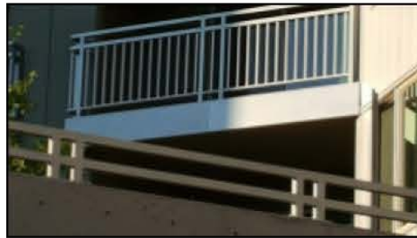
SILVER TONED RAILINGS AT ROOF DECK AND 2nd FLOOR TERRACES
