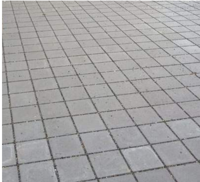
Permeable pavement
