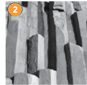
2 Concrete & Basalt Columns
