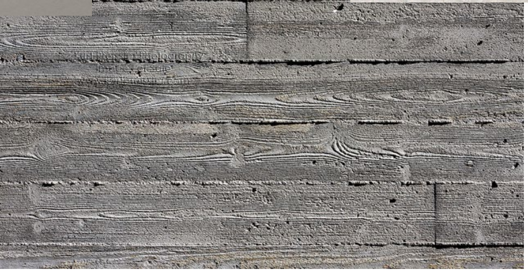
^ boardformed cast-in-place concrete
