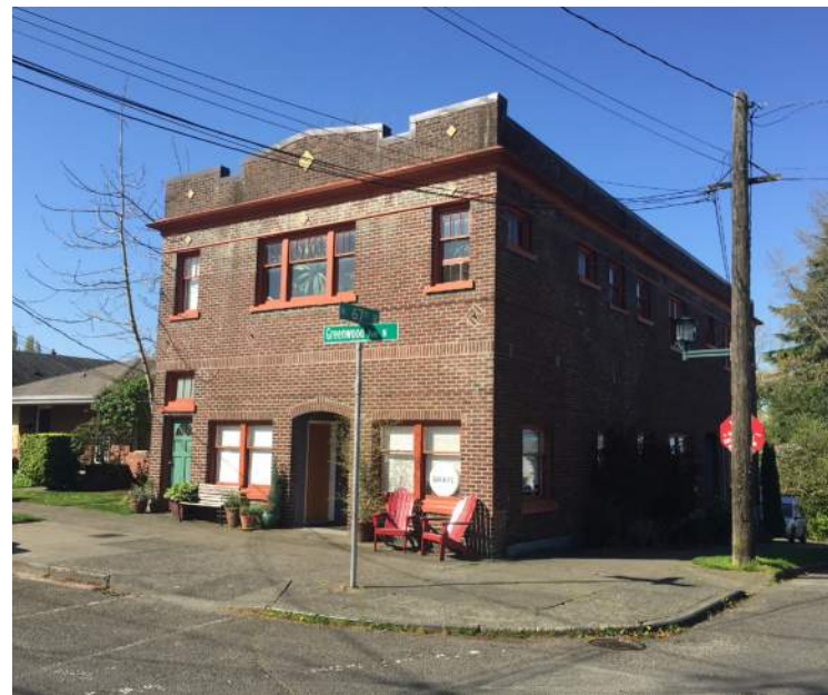
HISTORIC BRICK APARTMENT HOLD STRONG CORNER AND CONNECTION TO GROUND
