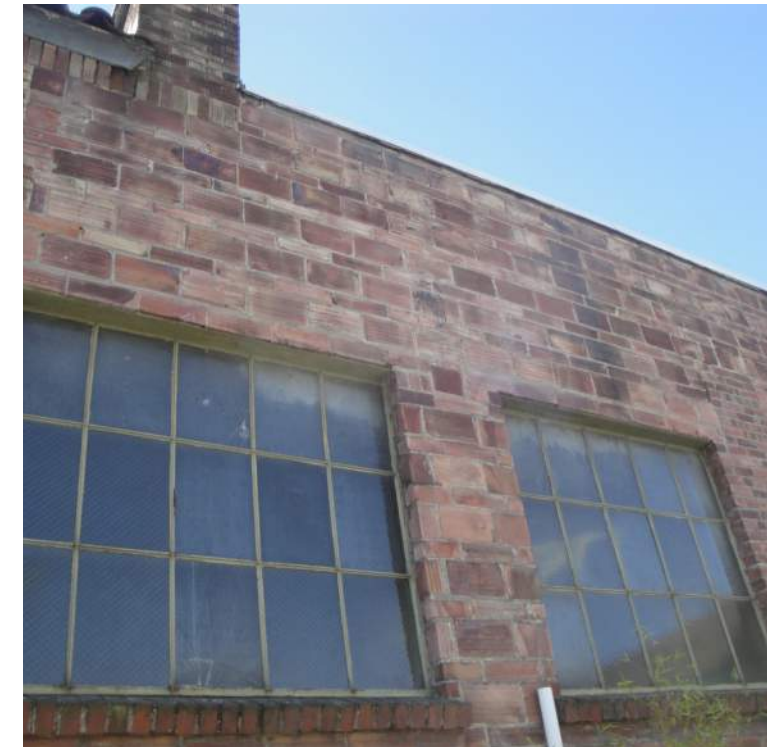
MASONRY FACADE WITH LARGE FRAMED OPENINGS
