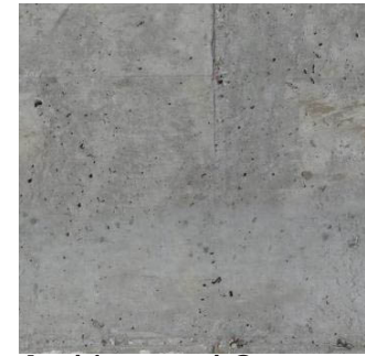
Architectural Concrete (AC)
