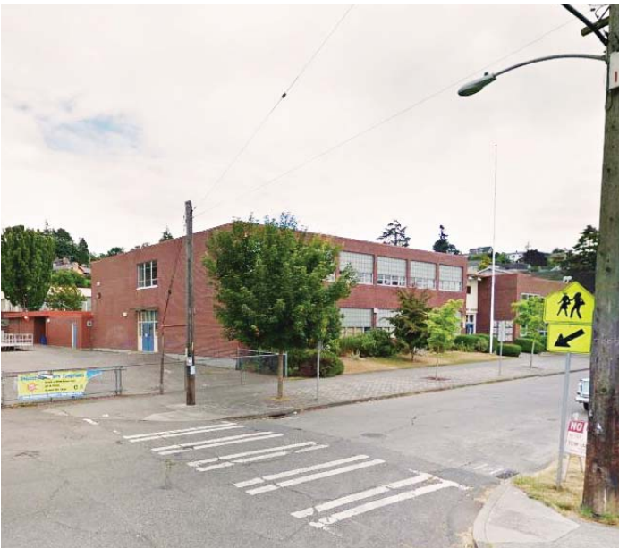
5 ALKI ELEMENTARY SCHOOL AT 3010 59TH AVE SW DISTANCE FROM SITE (0.5 MI): 🚲 2 MIN. 🚶 10 MIN.
