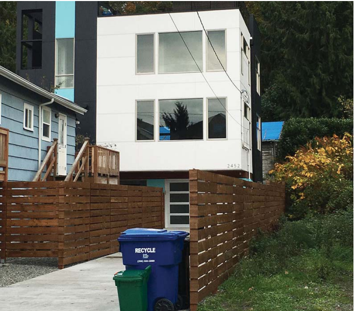
6 2452 55TH AVE SW SINGLE-FAMILY HOUSE
