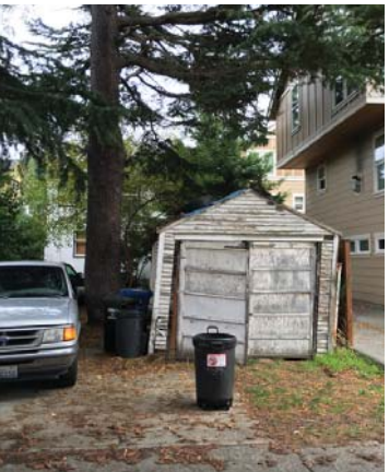
7 GARAGE TO BE DEMOLISHED
