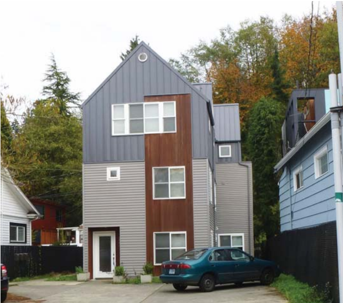
4 2446 55TH AVE SW SINGLE-FAMILY HOUSE
