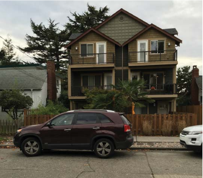
3 2425 55TH AVE SW TOWNHOUSE - NORTH OF PROJECT SITE
