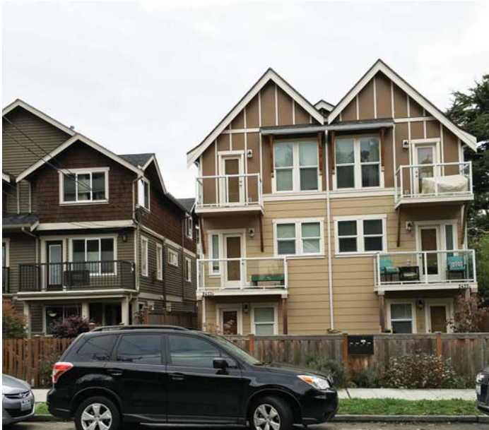
2 2433 55TH AVE SW TOWNHOUSE - SOUTH OF PROJECT SITE
