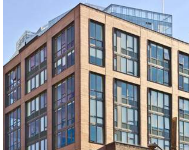
The Nolo Residential Apartments, Seattle, WA (Daniels Real Estate)
