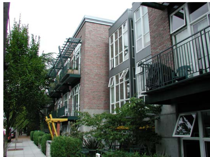
Metal Bays on Masonry on Queen Anne Driveway
