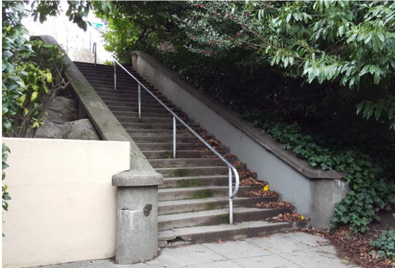
1. ACCESS STAIR-1st AVE W TO QUEEN ANNE DRIVEWAY
