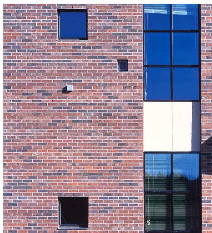
Brick and Punched windows on Queen Anne Driveway
