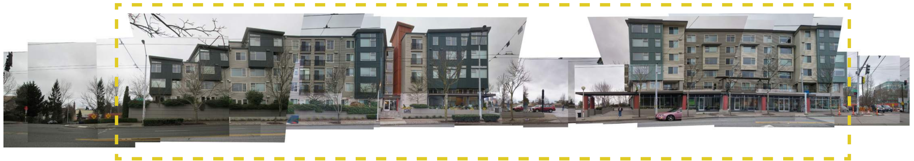
23RD AVENUE SOUTH - ELEVATION OPPOSITE SITE - LOOKING WEST
