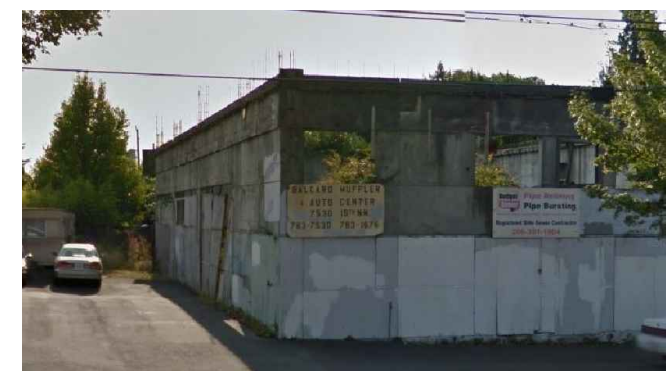
North facing facade on south muffler shop building
