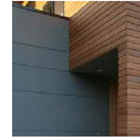
HARDIE PANEL AND WOOD CLADDING
