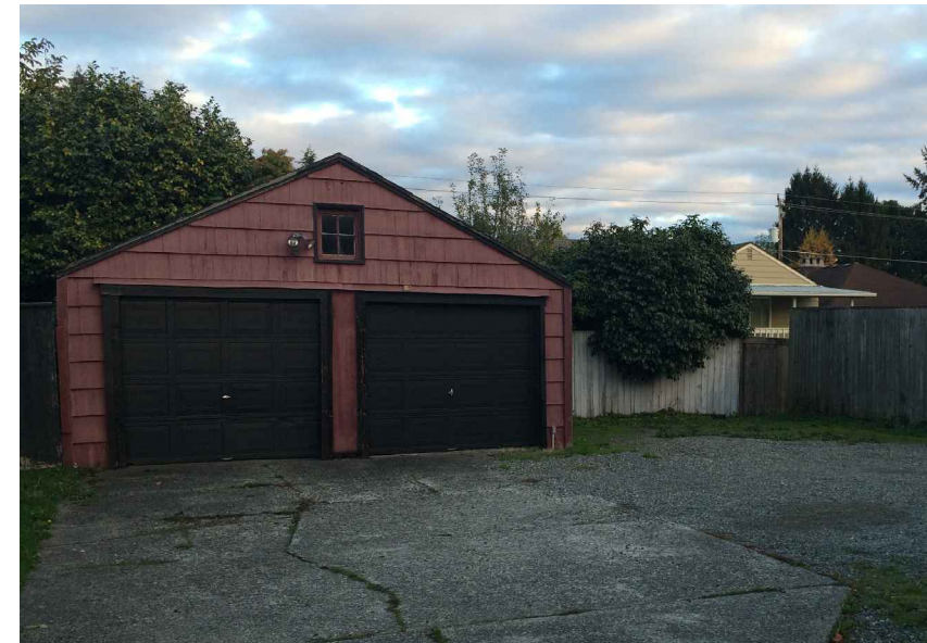
EXISTING GARAGE ON WESTERN EDGE OF SUBJECT SITE
