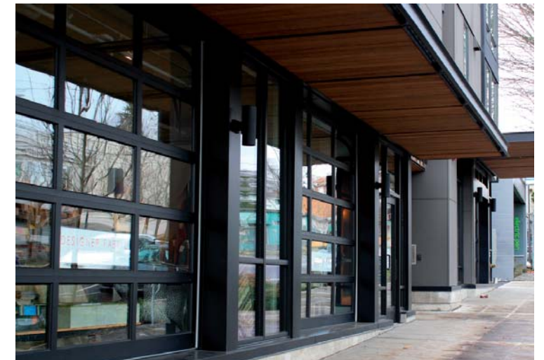
2 AWNING: WOOD AND STEEL AWNING ABOVE ROLL-UP DOORS
