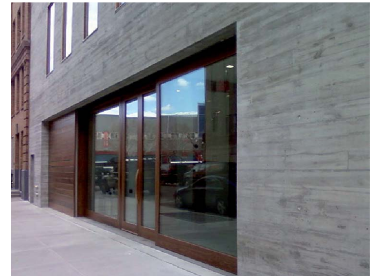
1 BOARDFORM CONCRETE AND GLAZING
