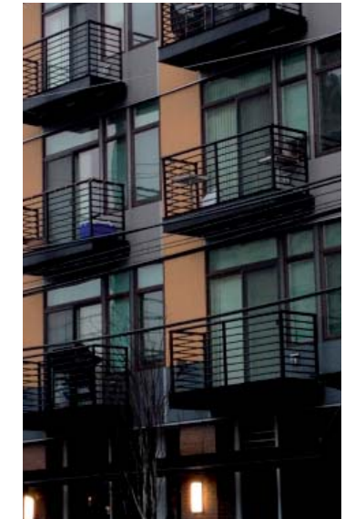
DECKS: STEEL OVERHANGS WITH ARTICULATED SUPPORTS
