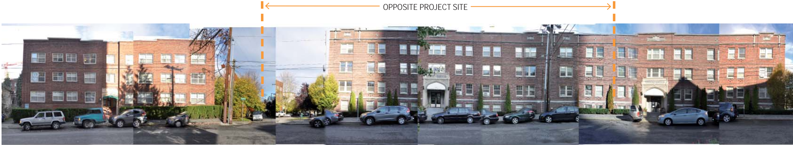
STREET ELEVATION A: E UNION ST LOOKING NORTH
