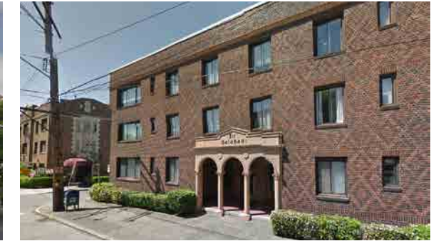
3- SIR GALAHAD 903 BELLEVUE PL E | APARTMENT This historic, 3-story, brick apartment complex is located directly south of our project site.
