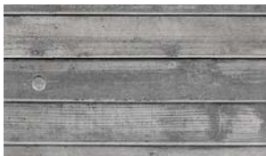
C1 Concrete Color: Natural Boardform Finish Use: L1 & L2 Exterior Walls
