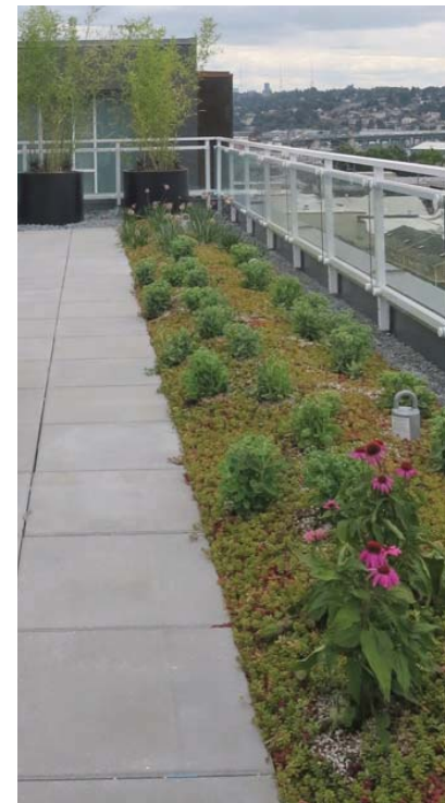
low landscape at guardrail
