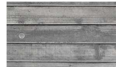
C1 Board Form Concrete
