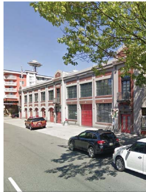
1 SEATTLE EMERGENCY MANAGEMENT 2320 4TH AVE
