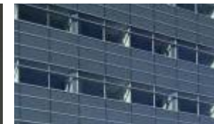
WW2 Window Wall w/ Tinted Vision & Spandrel Glass Insulated Clear Units / Opaque Glass Units Finish: Powder Coated - Iron Mountain Gray Use: Field Panels
