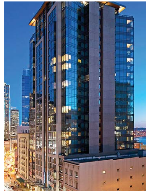
6 VIKTORIA APARTMENTS 24-STORY APARTMENT BUILDING
