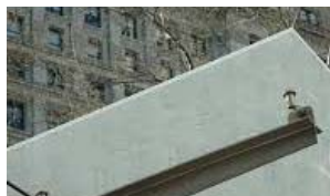
GL1 Glass Viracon - Frosted Use: Street Canopies
